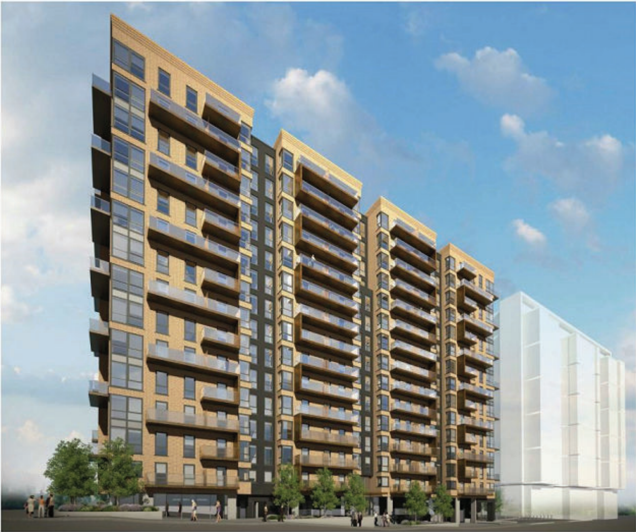
View looking down Rutherford Way
